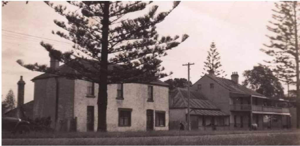
Figure 6. Port Macquarie Museum building, cottage at 24 Clarence St and Garrison Bldg circa.1940's.
